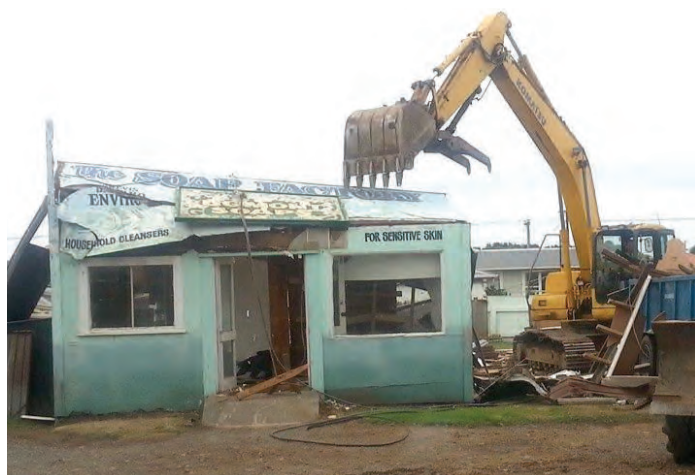
Egmont Soaps factory being pulled down recently.
