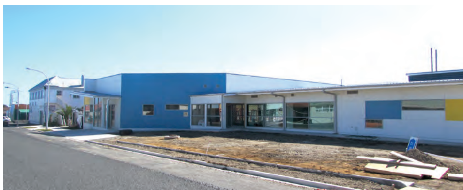
The front of the new Opunake health centre site is being tidied up, as the big opening day gets closer
